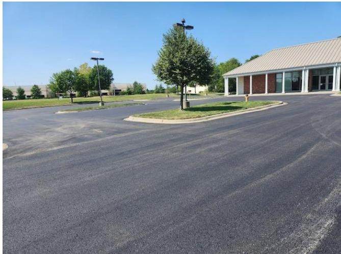
**Parking Lot:** The entire parking lot was completely repaved in August. This included replacement of curb areas that had cracked/deteriorated.
